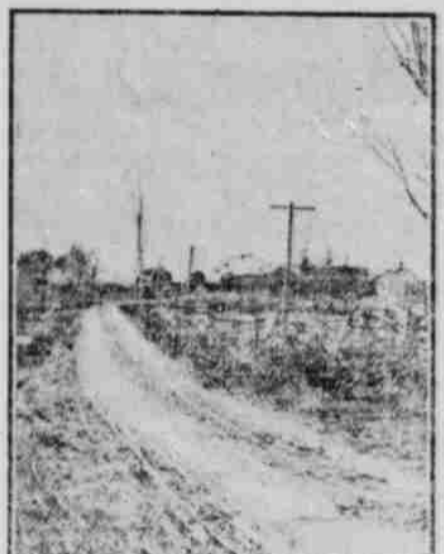
THE SAME ROAD MACADAMIZED.
