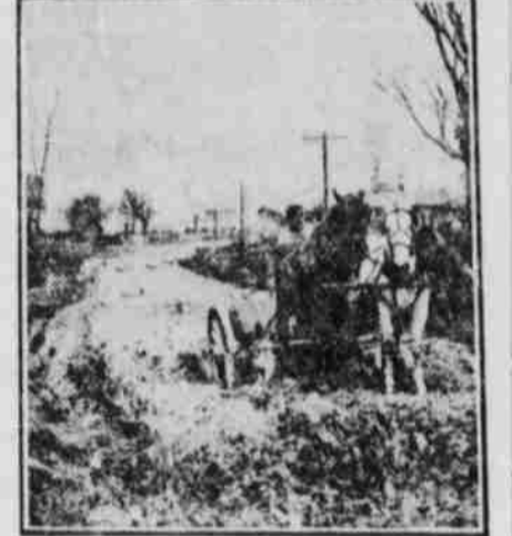
COUNTRY ROAD UNIMPROVED.
