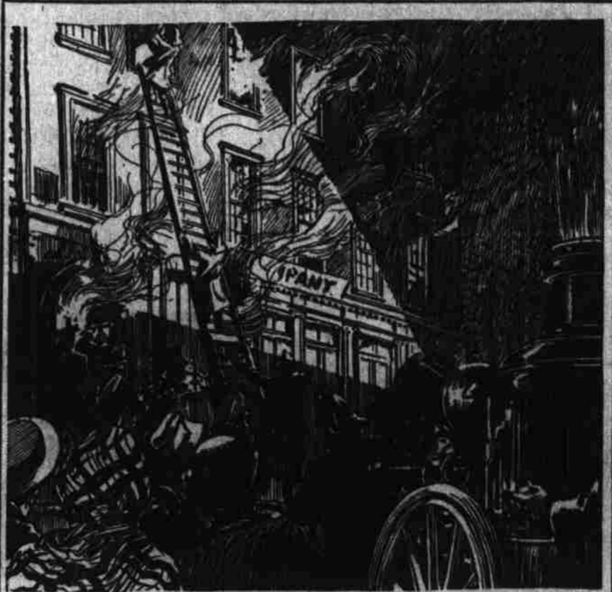
FIGHTING FIRE WITH AN ELECTRIC LIGHT. The New York fire department has just adopted and is making good use of the electric searchlight in fighting nocturnal conflagrations. A portable dynamo supplies the power for the light, which can be trained in any direction and is of especial use in combating fires in the high buildings that abound in Gotham.
