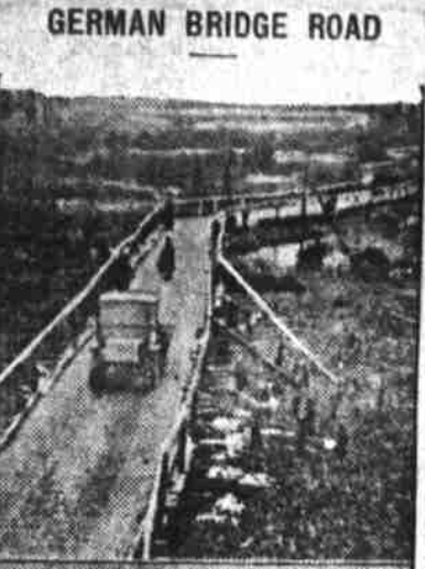
GERMAN BRIDGE ROAD Bridge road 546 yards long in northern France which was built by 600 German soldiers in five days.
