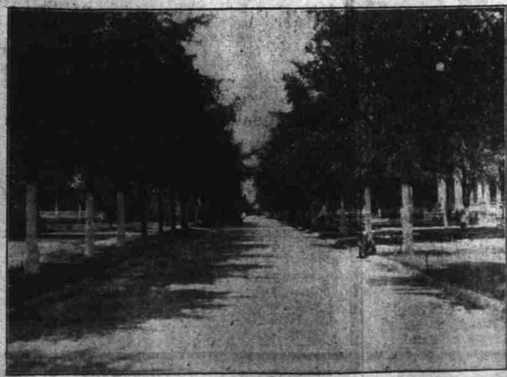
Evidence of one of Kinston's big steps forward. A street recently asphalted, one of many improved in a paving program that is costing the municipality and individuals between $400,000 and $500,000—Wide, shady, surface smooth enough to skate on.
