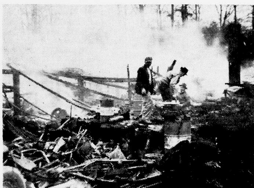
The above photo shows how completely the North State Auto Parts company building was demolished by fire here last week. Firemen fought the blaze for about five hours.
