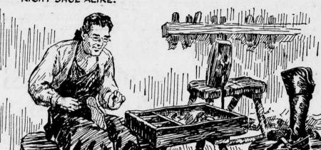
SHOE MAKING REMAINED A HANDICRAFT UNTIL 1815, WHEN THOMAS BLANCHARD, A NEW ENGLANDER, INVENTED A LATHE FOR PRODUCING LASTS. BUT IT WAS NOT UNTIL THE ADAPTATION OF ELIAS HOWES SEWING MACHINE TO THE STITCHING OF SHOES IN THE LATE 1840'S THAT THE BASIS OF THE MODERN SHOE MANUFACTURING INDUSTRY WAS ESTABLISHED.
