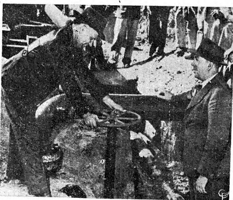
DISTRICT SUPERINTENDENT Tom Evans (left), of the Tennessee Gas and Transmission Company, and R. W. Hawkins, divisional superintendent, are shown opening the valve on the company's main transmission line at Natchitoches, La., which carries natural gas at a rate of 50 million cubic feet daily into the "Little Big Inch" pipe line. The gas is being pumped to the middle west, where it will help alleviate the fuel shortage brought on by the current soft coal walkout. (International)
