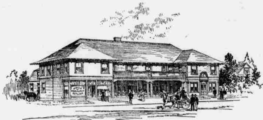
PINEHURST'S NEW DEPARTMENT STORE BUILDING.
