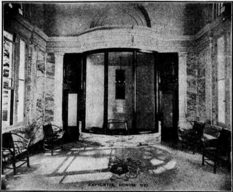
INTERIOR VIEW OF NEW SPRING HOUSE.
