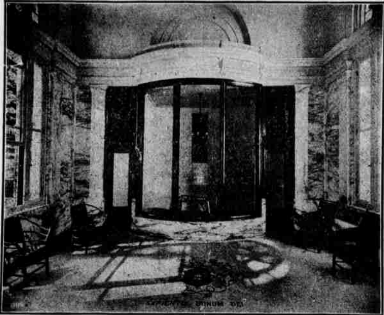
INTERIOR VIEW OF NEW SPRING HOUSE.
