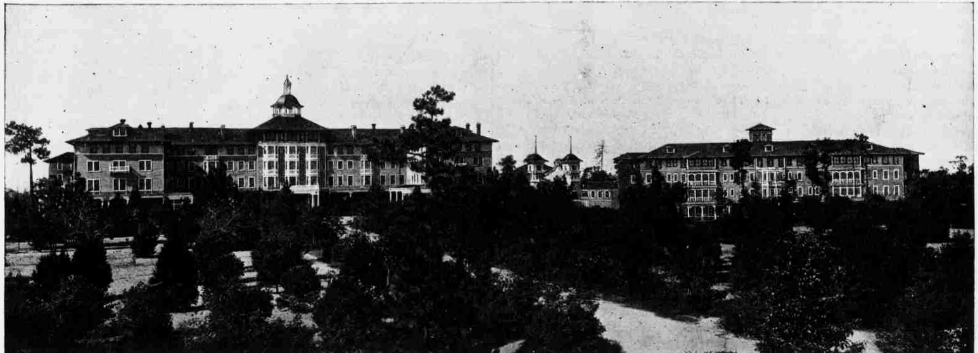
THE SEVENTY-ROOM CAROLINA ADDITION CONTAINS SIXTY-TWO BEDROOMS, EACH WITH PRIVATE BATH, AND SIXTEEN SLEEPING PORCHES
