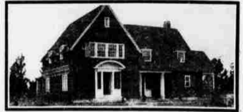
WEYMOUTH HEIGHTS, Southern Pines, North Carolina On the main line of the Seaboard Air Line, sixteen hours from New York. A residential community, well located, with Southern exposure and extensive view, clustered around the Highland Pines Inn. Ten minutes' walk from the center of town; five minutes' walk from the Golf Club.
