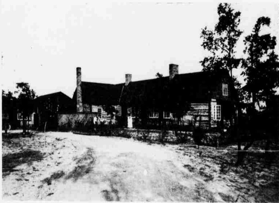
THE BUTLER HOMESTEAD IS IN HARMONY WITH THE COUNTRY
