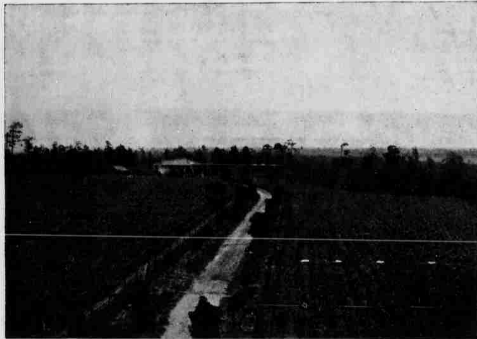
APPROACH TO THE PUMPELLY HOUSE AT SAMARCAND
