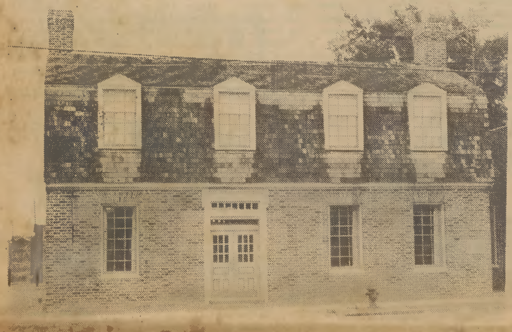
The Farmers Bank of Seaboard Building
