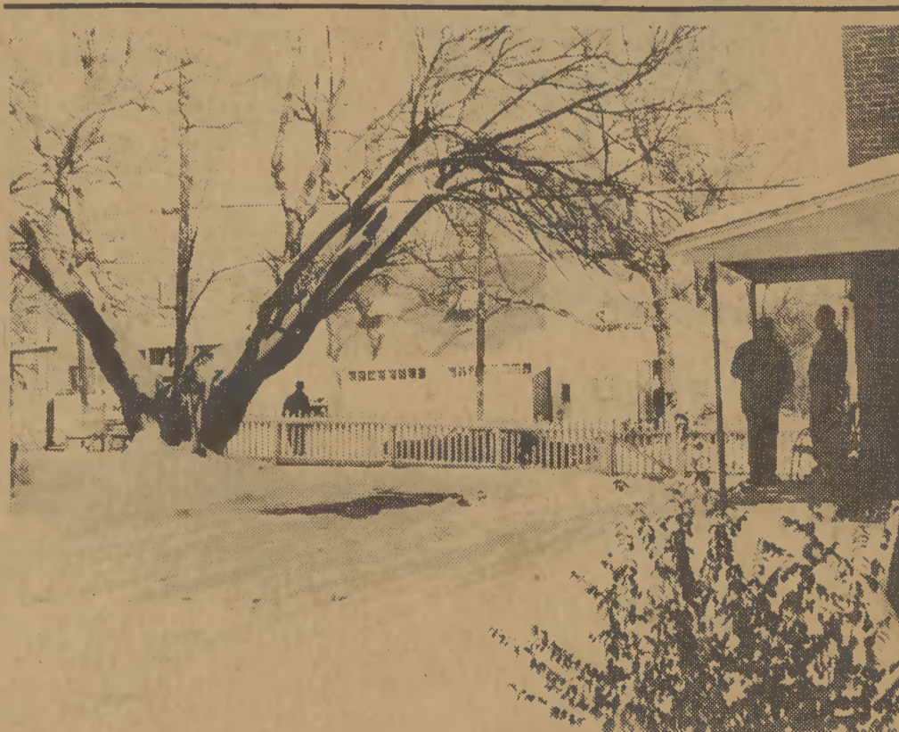
RENOVATION OF THE COUNTY JAIL, which should begin early next month, will include the extension of the building from its present location at right to a point 22 feet (next to the tree) at left. County Accountant Tim Ellen and County Jailer John Cox are almost silhouetted against the bright outdoors as they survey the proposed work. Ellen said that the delay in starting the work was centered around delivery of the materials. The contractors have 240 days from November 6 to complete the job.
