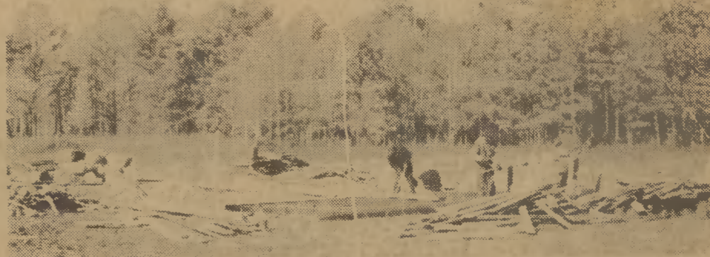
THIS SCATTERED LUMBER WAS HOME for two horses until a small "twister" touched down briefly in Rich Square during the severe weather last Friday afternoon. The stable, owned by Dr. B. E. Stephenson, a Rich Square physician, was located on Bryantown Road. The two horses were not injured so it is assumed they were outside in the corral when the wind struck. Other minor damage was reported in the area, including a downed antenna and the uprooting of a tree. Tuesday, when this picture was taken workmen were busy cleaning up the damage.
