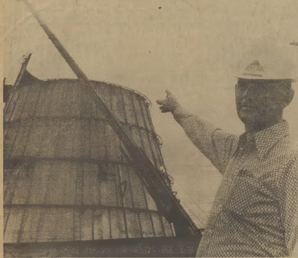
COMING DOWN — Willie Duke, general plant manager, of Georgia-Pacific in Conway gestures towards the plant's tee pee or conical waste burner that has been the source of a pollution problem at the plant. The burner will be replaced eventually with a modern boiler that will be fired from the plant's waste matter. In the interim the plant will operate a sanitary landfill to handle the solid waste.
