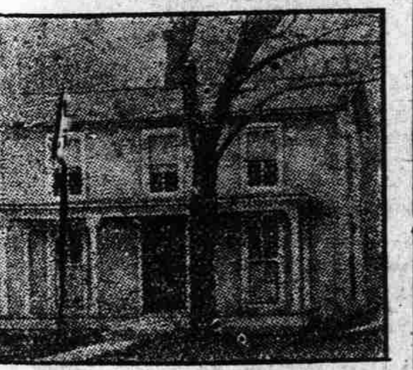
BIRTHPLACE OF W. J. BRYAN, AT SALEM, ILL. (On this site a library will be built to mark the spot in the future.)
