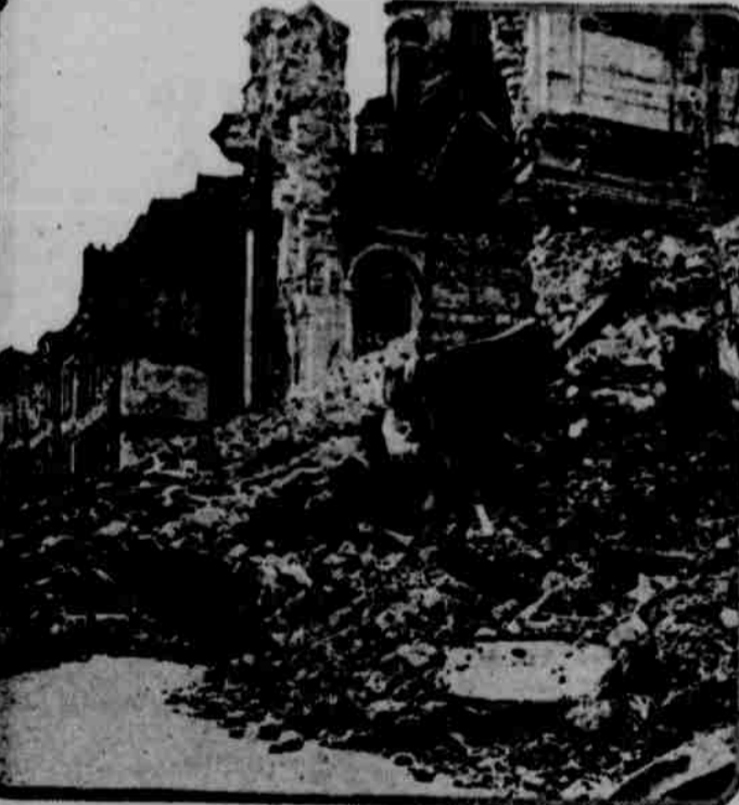
Nothing was spared by the Germans in their ravages in French towns. Beautiful cathedrals were wrecked irreparably. Almost every home is a mass of debris. When the British entered Arras they found this inconceivable mass of ruins. The picture was taken outside the wrecked cathedral.
