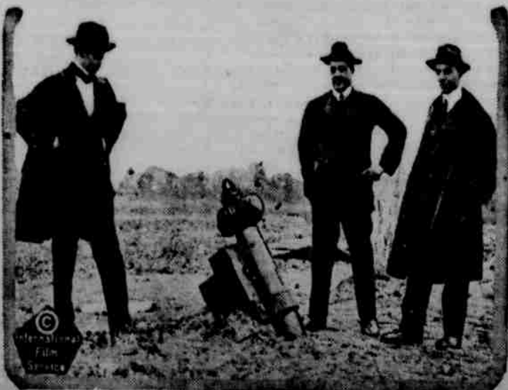
Here is a new kind of a mortar. Instead of throwing shells it throws barbed wire. It can throw five rolls of barbed wire into enemy trenches or in front of advancing troops without being recharged.
