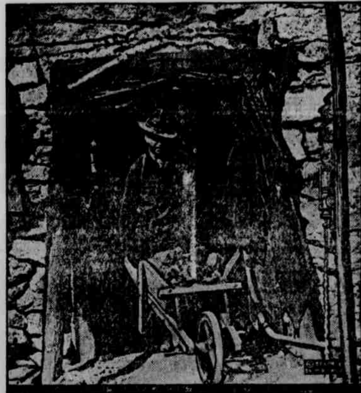
American engineers are doing splendid work in extending and perfecting the trench system in the American sector in France. Demolished walls and ruined buildings are considered especially valuable for the establishment of intermediate depots and posts. This American engineer is converting a tunnel into a post command by the quick methods known to army constructors.
