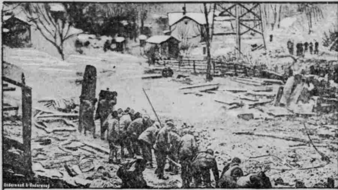
Men fighting a gas well fire at Snake Hollow, just outside McKeesport, Pa., where vast quantities of natural gas have been discovered recently. The men with the long pipe are trying to knock the cap off the well so the fire can be extinguished with steam.
