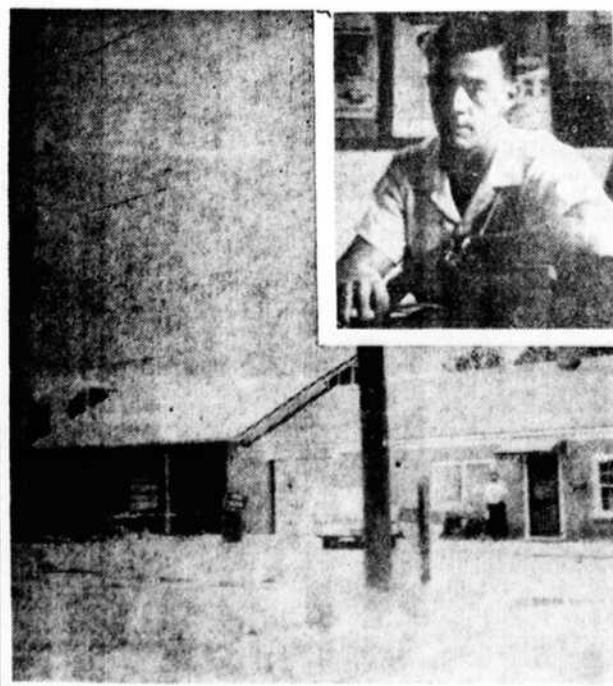
VOLUNTEER LABOR and contributions from merchants and friends of the Fair Bluff Fire Department will make the construction of a new fire house possible, with completion expected by the end of the year. The new chief, Carwell Hughes (inset), said that his men are very grateful for the backing given the squad by the citizenry for this project, as well as for the acquisition of a rescue and emergency truck. Fair Bluff aldermen have also ordered a new fire truck.
