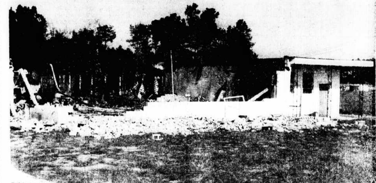
DESTROYED BY FIRE — Shown is what was left after the fire Thursday night which gutted Cox Brothers furniture plant. At the right is the iron works which was saved. (Staff photo)
