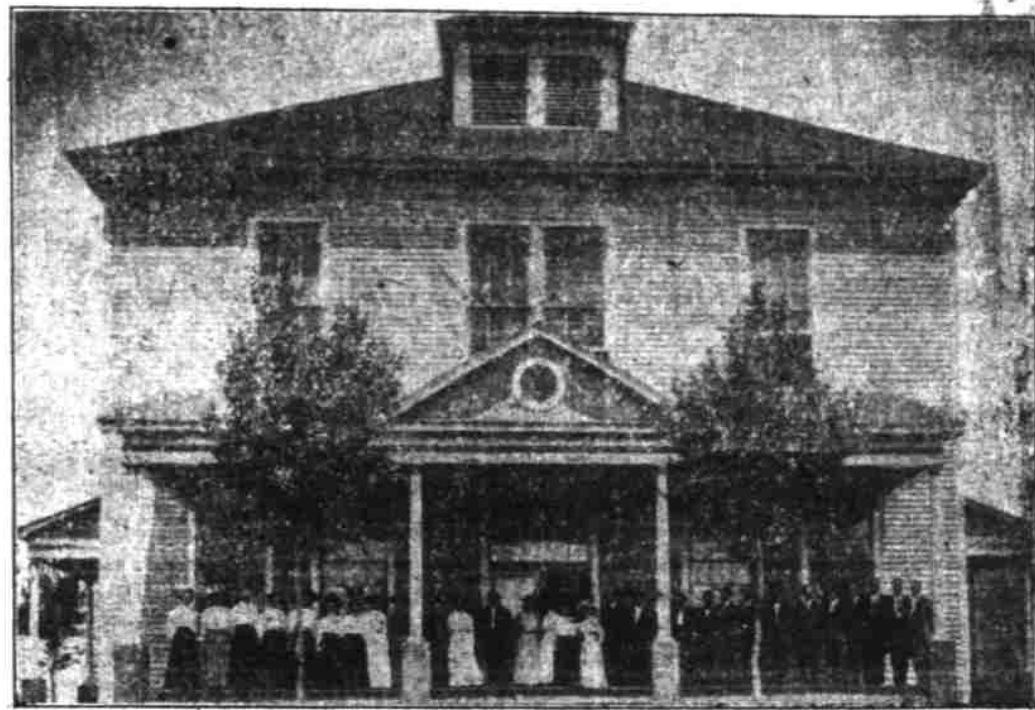
WEBSTER HIGH SCHOOL BUILDING
