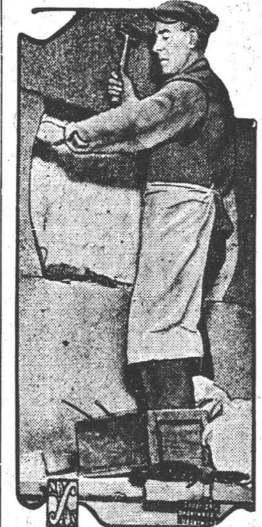
Albert Beer, stonecutter for twenty-five years, is seen tearing a hole in the side of the Washington monument in the capital to make ready for another of the inscribed state slabs. This one will be a slab of petrified wood from the state of Arizona.
