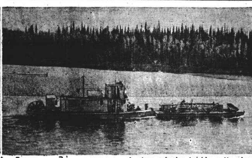
A stern wheeler briskly puts along Dease Lake, transporting construction equipment by barge to the Watson Lake airport. In shallow waters of the Stikine River boat crews had to remove rocks to make passageway for these crafts.
