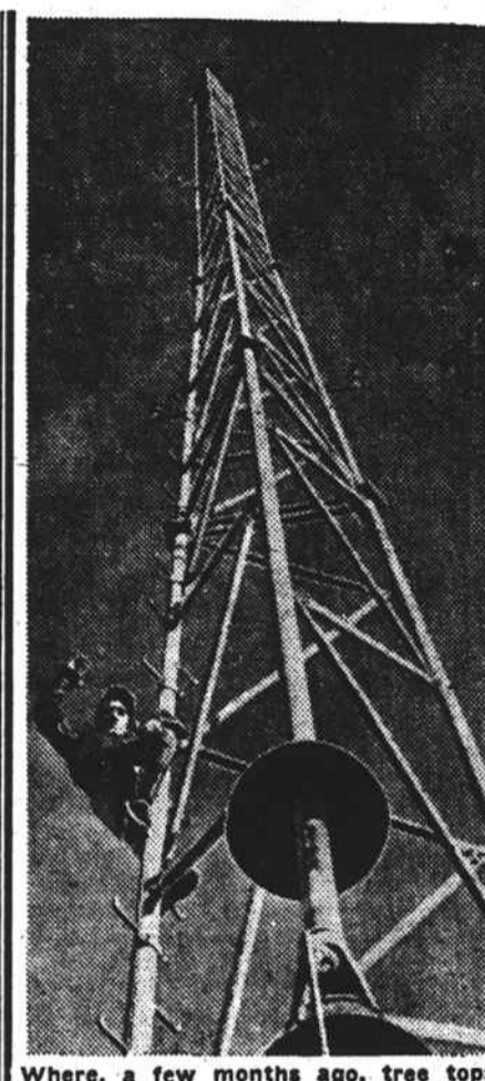
Where, a few months ago, tree tops filled the sky, wireless towers stand to guide planes on the new Alaska air route.
