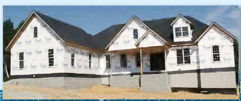
Under Construction - Custom Built Energy Star Home with Solar Panels
