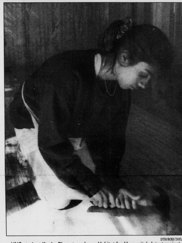
UNC student Kanku Bhagat works on Habitat for Humanity's latest project.
