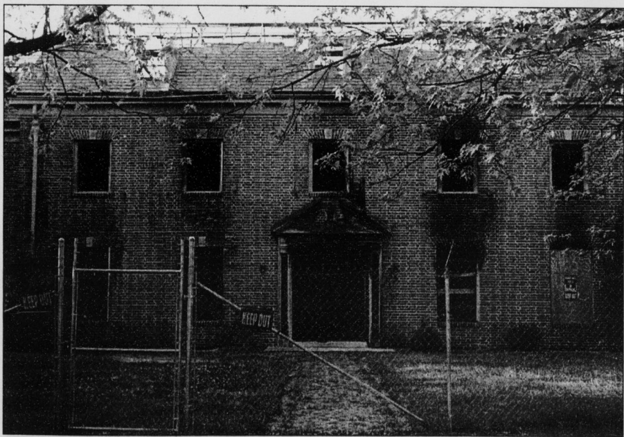
A fire killed five UNC students in May 1996 at the Phi Gamma Delta fraternity house. This incident caused the N.C. General Assembly to pass a new law that requires sprinkler systems be installed in all fraternity and sorority houses.
