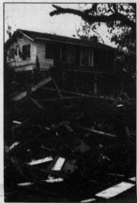
A home in Mississippi shows the devastation produced just after Hurricane Katrina, which hit the Gulf Coast one year ago Tuesday. DTH FILE PHOTO
