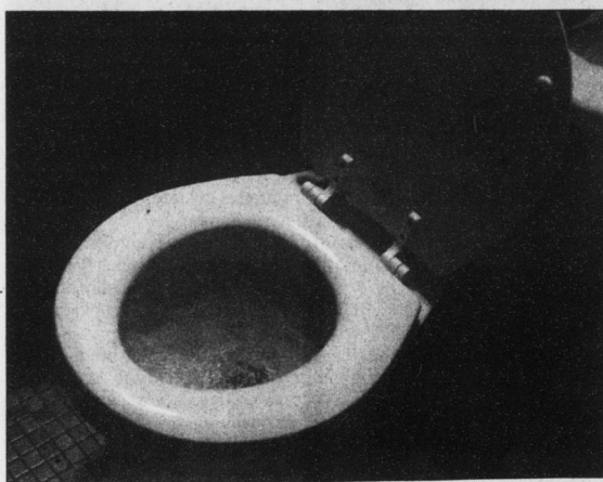
Cedar Court just installed new low-flow toilets that use 1.6 gallons of water instead of 5 gallons. Cedar Court residents support the idea.
