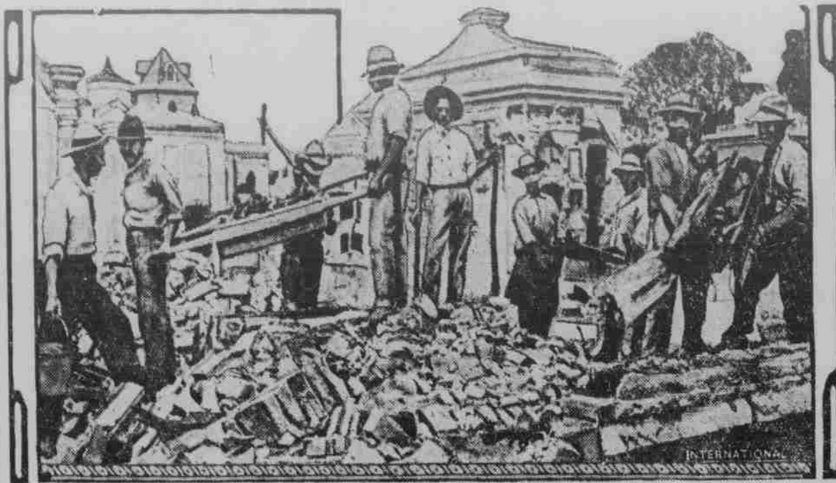
This is the first photograph received from San Jose, Costa Rica, since the disastrous earthquake. It shows men at work in the Heredia cemetery, where many of the burial vaults were reduced to ruins and numberless bodies were unearthed by the temblors.
