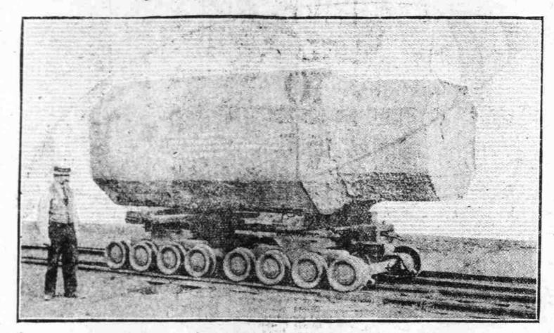
Greatest of its kind is the gigantic steel; ingot, weighing 90 2-10 tons, from which was made the breech end of the great 16inch gun which has just been bored and rifled at the Watervilet Arsenal. The ingot was Works, and is the largest piece of solid steel ever east in the world.
