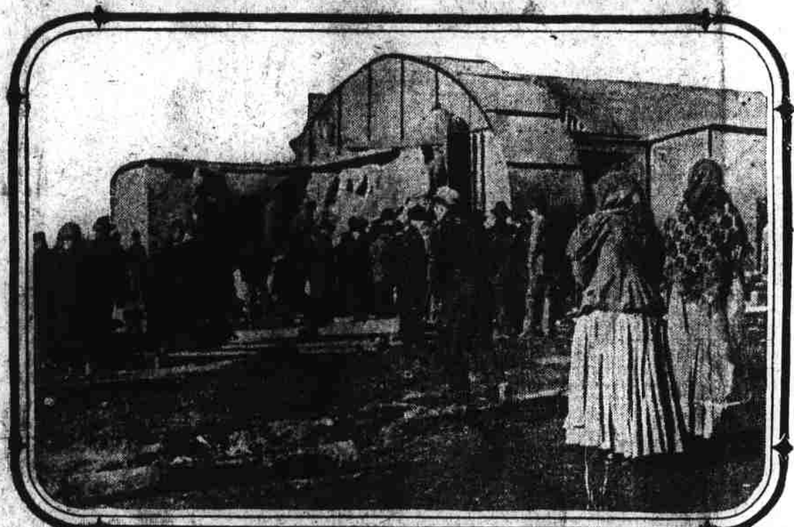
Scene at the mine in Cherry, Ill., as rescuers prepare to descend to look for bodies of the entombed.
