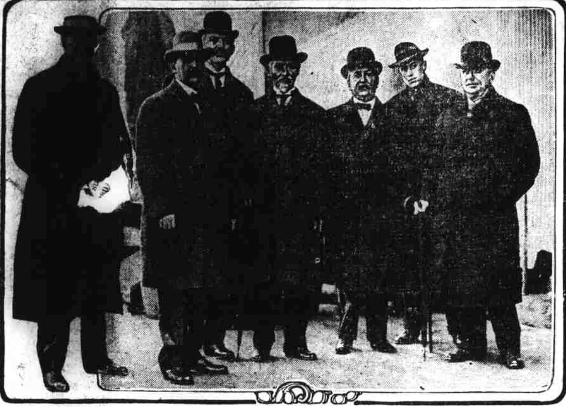
The Committee on Appropriations of the House of Representatives, which has returned from Panama, where it had been inspecting the canal. The several members are enthusiastic over their trip and unite in saying the work is progressing in splendid fashion.
