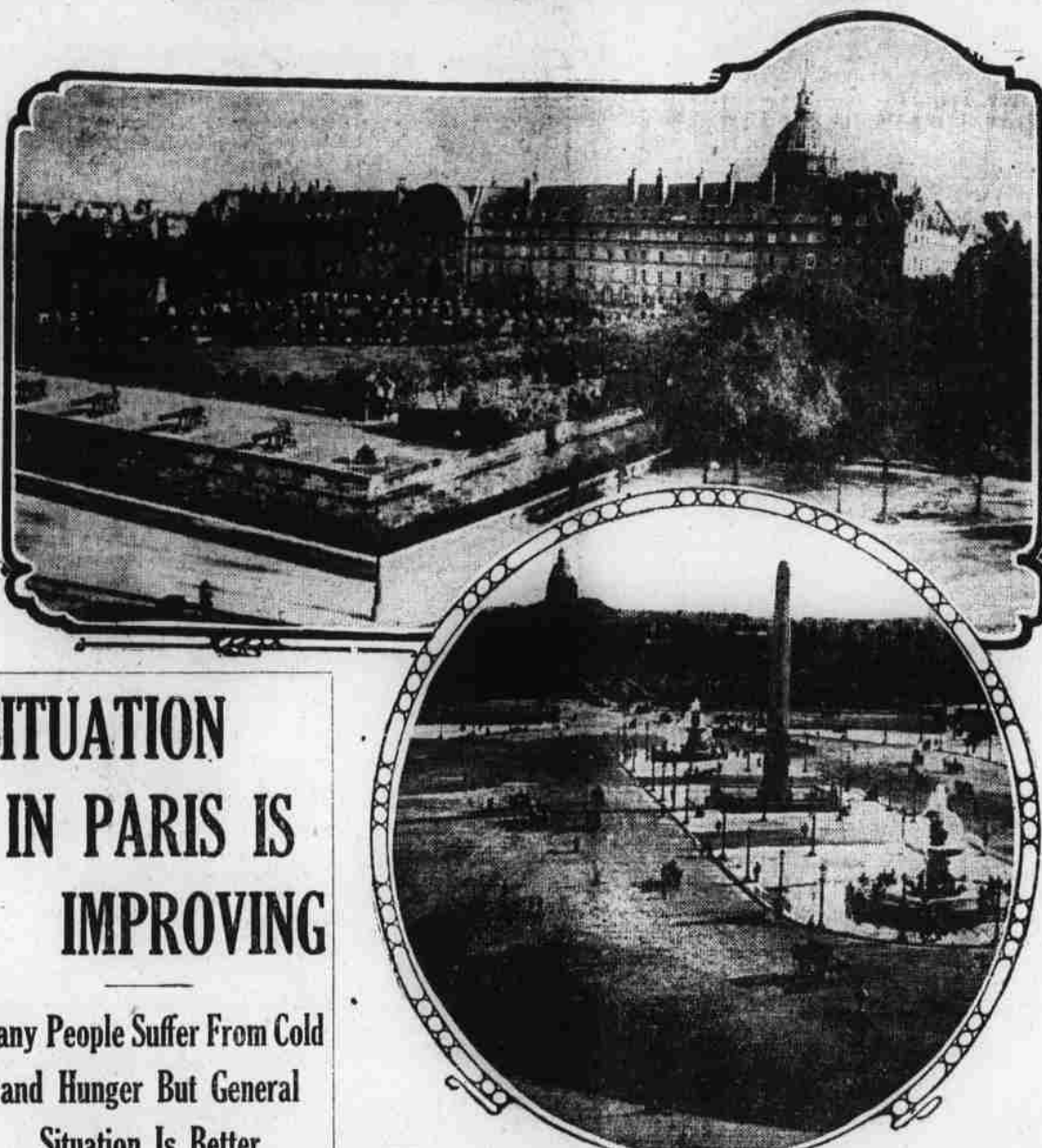
The Hotel des Invalides, in Paris, which for several days past has been surrounded by water because of the recent floods. The lower picture on the right shows the Place de la Concorde, which has been completely flooded. Both of these views are of places and buildings in the very heart of Paris.
