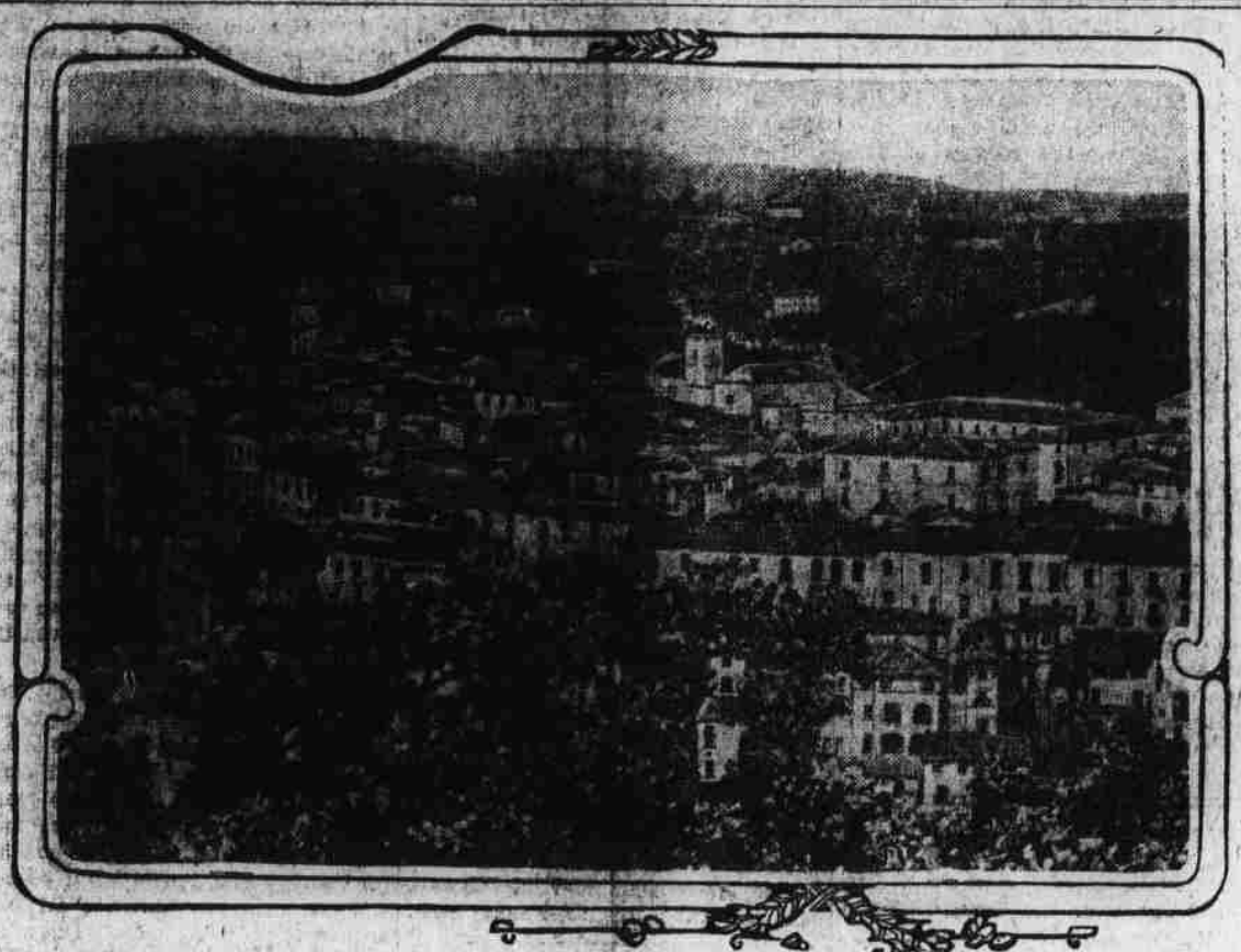
Panoramic view of Asheville, where the earthquake of June 7th is reported to have done much damage. Nearly every house in that city and vicinity was thrown down by the shock. At least fifty persons were killed according to the meagre reports from the scenes of the disturbance.
