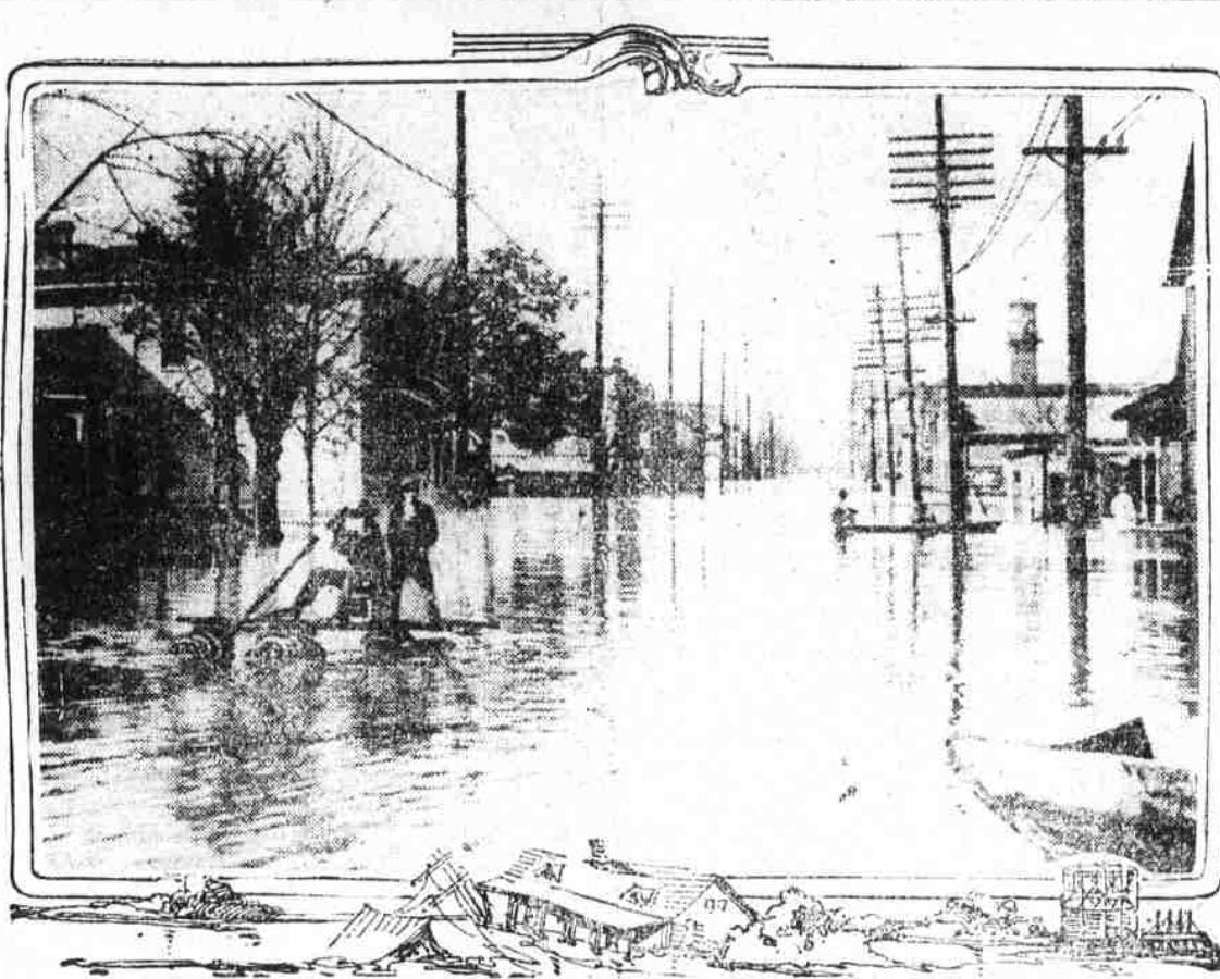
FLOODED SECTIONS OF MEMPHIS. The photograph shows the condition of a street running parallel with the river, but two blocks from the water front.
