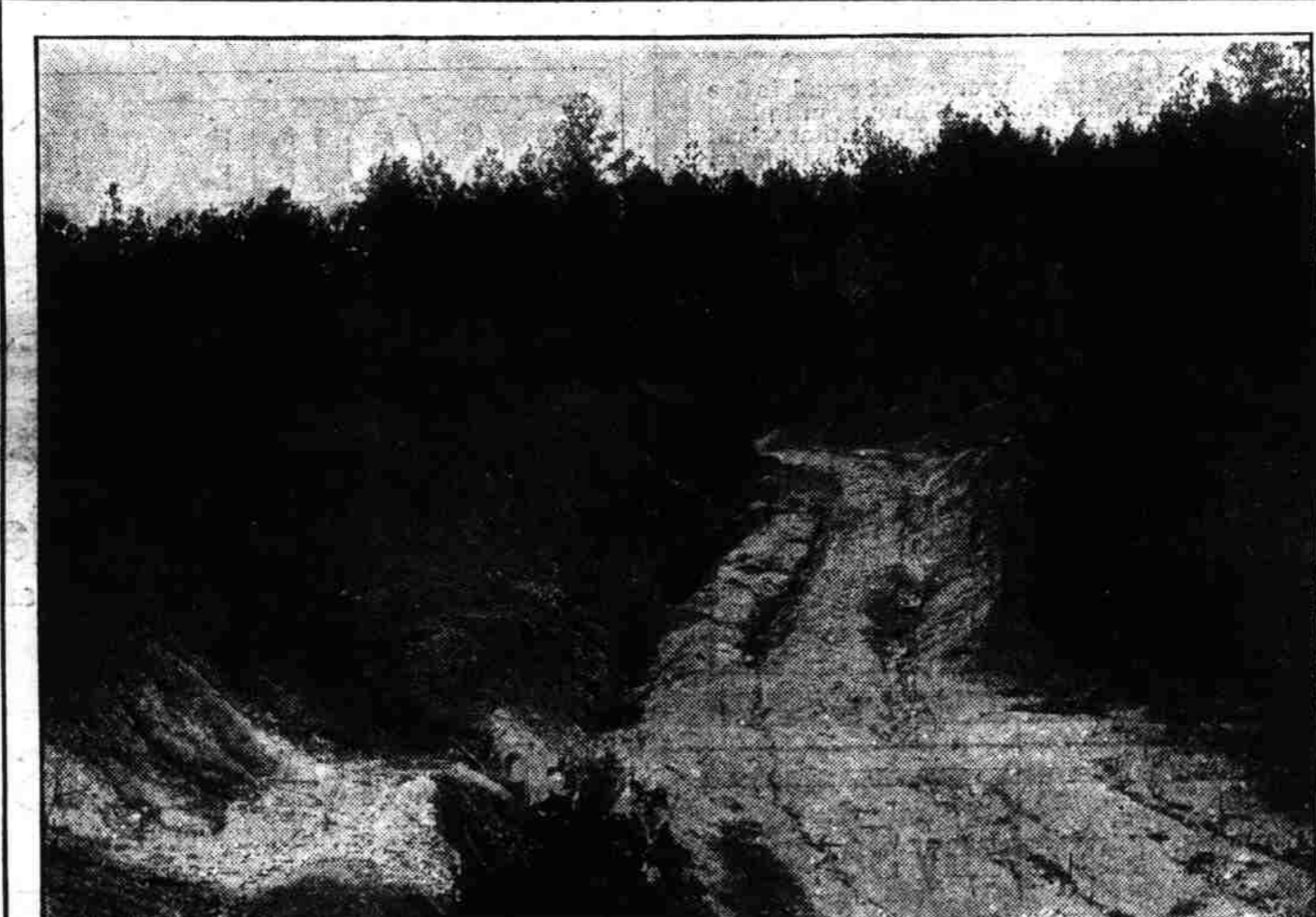
NOTE HOW THE SOIL OF THE FIELD IS BEING WASHED DOWN INTO THE OLD ROAD-BED. THERE ARE THOUSANDS OF SUCH OLD FIELDS IN THE SOUTH.
