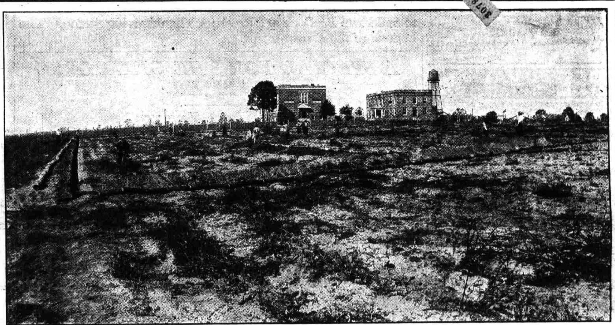
STUDENTS AT STATE AGRICULTURAL SCHOOL, MAGNOLIA, ARK., LAYING TILES FOR UNDER-DRAINAGE.
