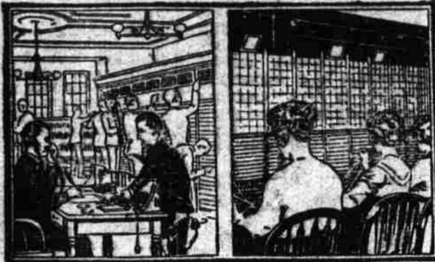
Early Telephone Exchange
