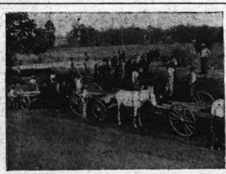
HAULING CLAY TO MIX WITH THE SAND
