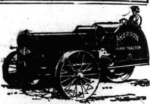
A four-cylinder, 2-speed, light-weight tractor of great power, suitable for any size farm. Will pull the implements you now have on your farm—gang plows, harrows, mowers, binders, manure spreaders, road drags or graders. Will also operate your ensilage cutter, feed grander, circular saw, etc Does more work than horses—costs less and is so simple anyone can run it. anyone can run it.
