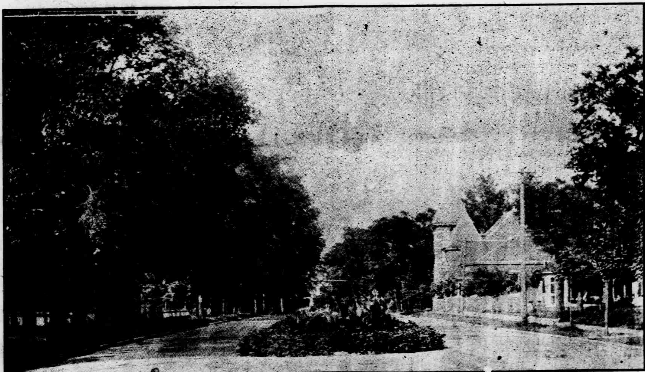
SPRING STREET LOOKING WEST
