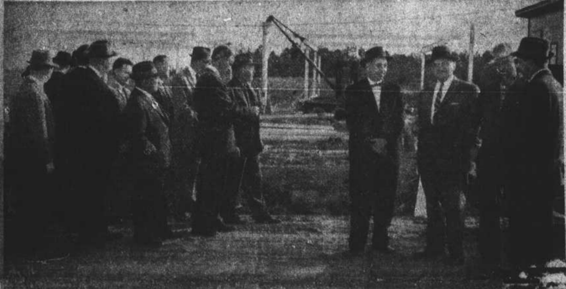
CONSTRUCTION SITE VISITED —Granville County business leaders are shown during a visit last Wednesday afternoon to the site of a shell factory building being erected by Granville Developers, Inc. on a 15-acre site west of town. J. P. Harris, Jr., a director of Granville - Oxford Planning Commission, W. T. Yancey, Construction Superintendent C. M. Hamlet of George W. Kane, Inc., and Louis Hutchinson, president of Granville Developers at right, discuss progress on the contract. The group later visited the Tobacco Station. —J. B. Clay photo
