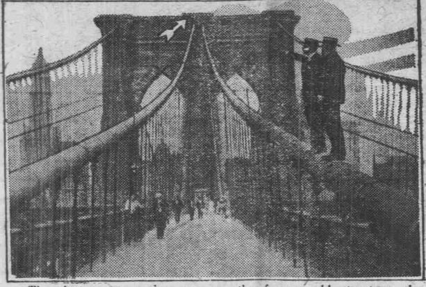
That largest suspension span on the famous old structure, the Brooklyn Bridge at New York, has slipped under the constant hammering of traffic and authorities have closed it to all except pedestrians. Arrow points to slipping cable,
