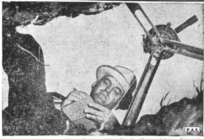
Here's a worm's-eye view of an avalanche in the making. Lowering himself into a huge fissure at the top of the "moving mountain" in Los Angeles' Elysian Park, a daring cameraman shows how the ever-widening crack is being checked hourly to determine course and extent of the next in a series of huge earth-slides that have already sent millions of tons of rocks, earth and trees tumbling 350 feet into Riverside Drive, Dayton Avenue, below, and even into the dry bed of the Los Angeles river, 1,000 feet away.
