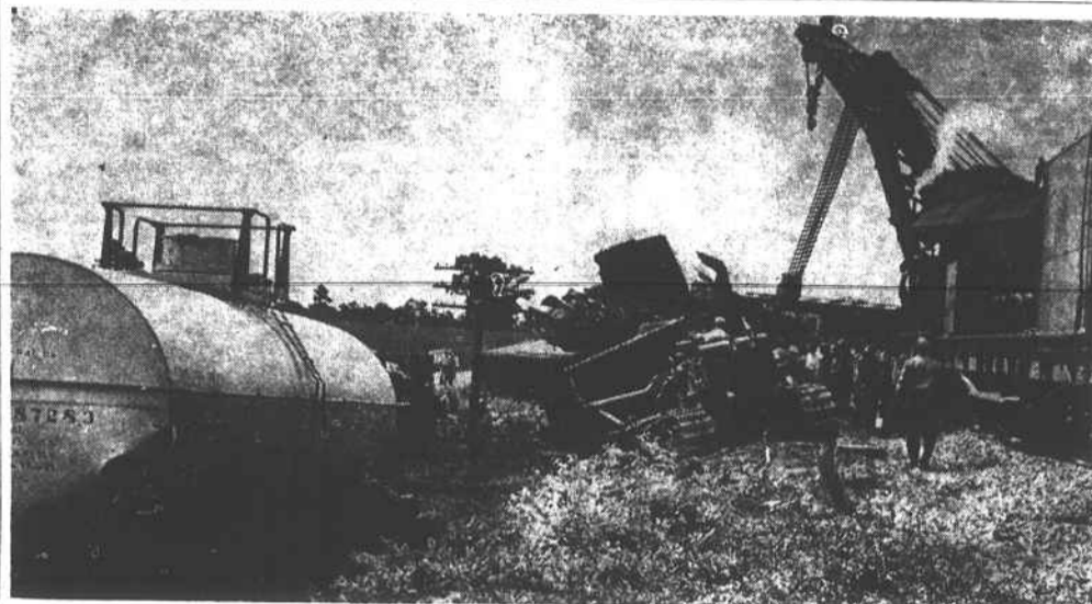
A large railroad crane is shown removing cars and wreckage from the lines of the Seaboard Air Line Railroad Company near Paschall on Saturday morning. Trains are running but much of the debris remains on the right-of-way. (Photo through courtesy of The Henderson Daily Dispatch)
